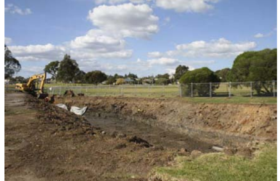
Preparing for installation of the reserve wastewater storage tank
