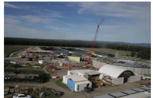
Gippsland Water Factory Construction site - June 12, 2008
